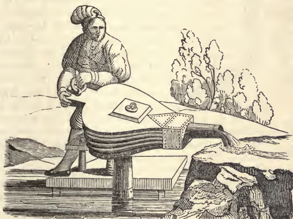
No. 82. German Atmospheric Bellows Pump. A. D. 1511.
